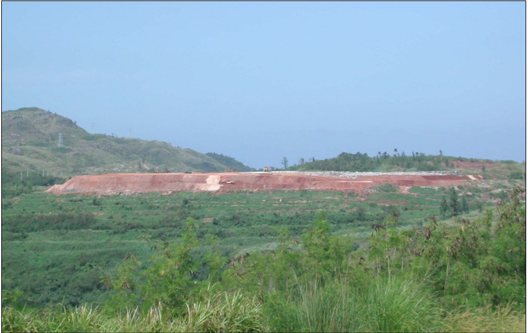
Ordot Landfill looms over the Lonfit River valley where it occupies ~60 acres of land space and towers upwards to a height in excess of 90m at its mid-point (2003 photo: courtesy Leroy Heitz, WERI)
