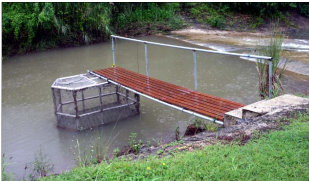
Figure 28: Picture of the Ugum River Treatment Plant's intake structure
