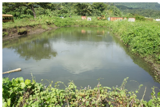
Figure 14. Third oxidation pond.
