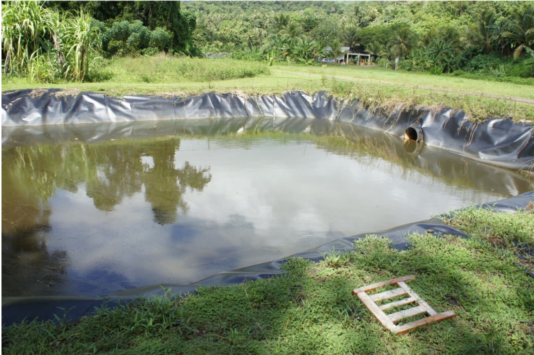
Figure 4. Lined leachate catch pond at the landfill on Kosrae. Image source: author.
