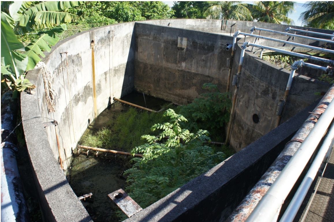
Figure 7. Inoperative sewage treatment plant on Weno Island in Chuuk state.
