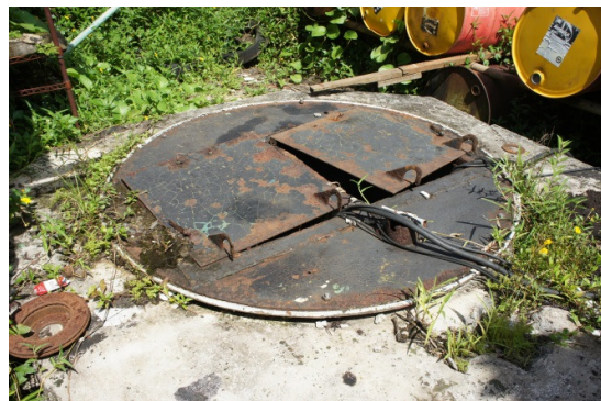
Figure 20. Collection pit for septic tank effluents in Lelu Village.
