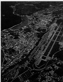
Figure 7.1. Guam International Airport and runway complex. (Courtesy: GIAA)
