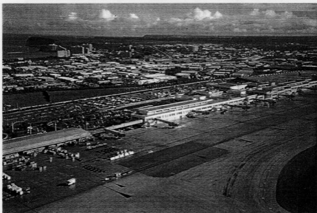
Figure 7.2. Guam International Air Terminal from runway side showing jet ways.
