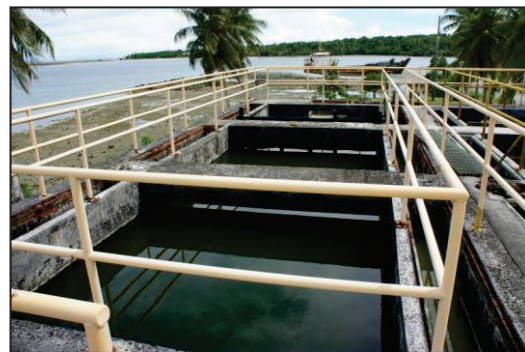
Interior of the Yap Sewer Plant
