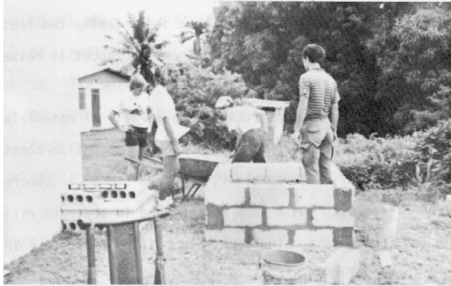
Figure 3: Block Tank Base
