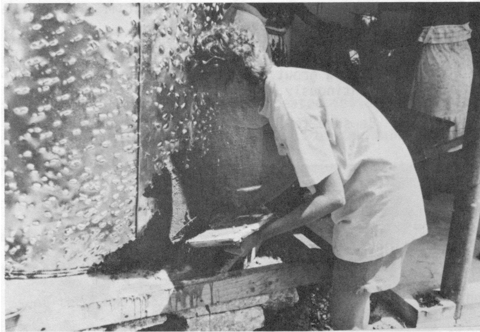
Figure 16: Grouting
