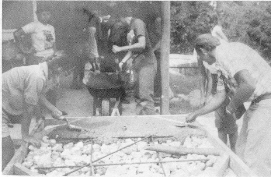
Figure 14: Concrete Slab
