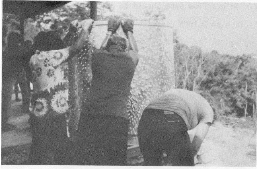
Figure 9: Shell Installed into Slab
