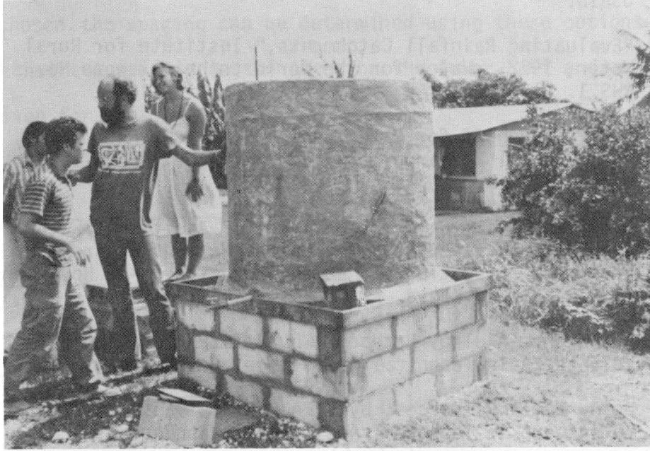
Figure 20: Water Storage Tank
