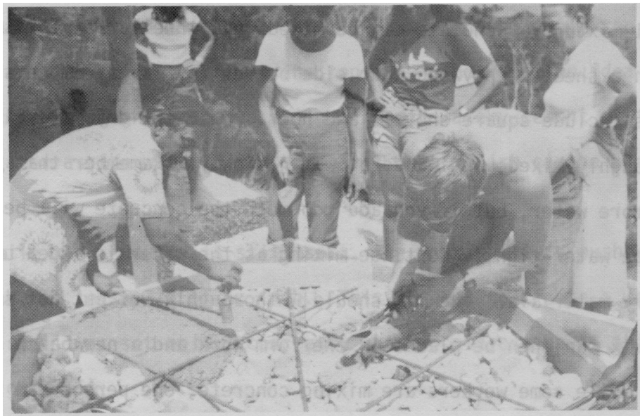
Figure 13: Preparing the Piping
