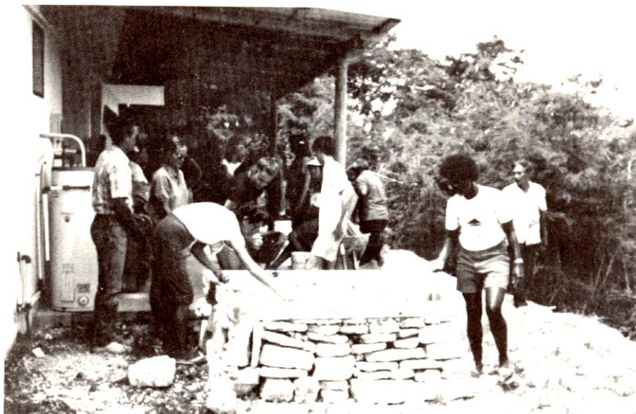
Figure 2: Stone Tank Base
