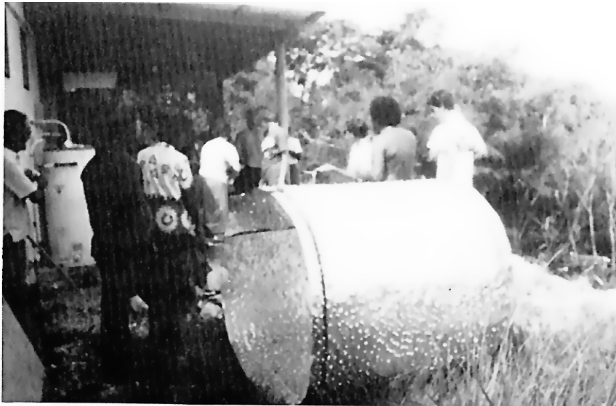
Figure 8: Shell is ready for Installation
