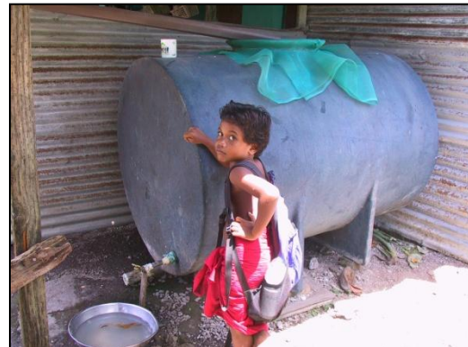
Rain water storage tank in the FSM.
