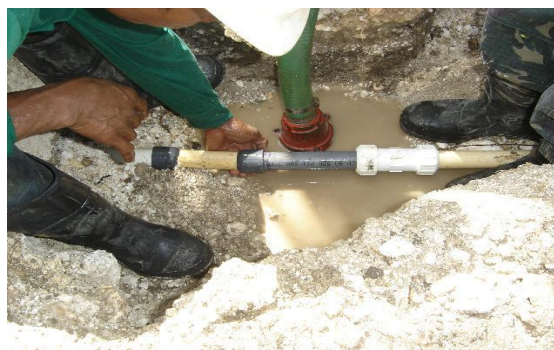
WERI Leak Detection – Saipan 2011
