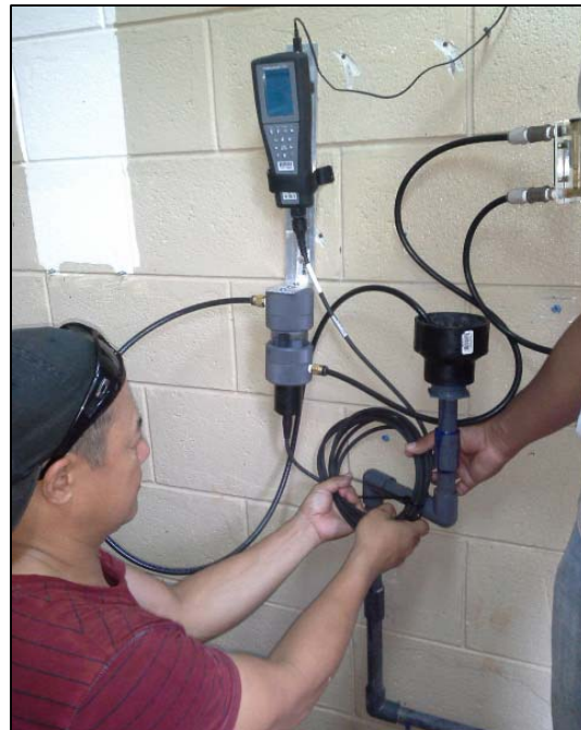
Installation of multiprobe meter at GWA well F-13.
